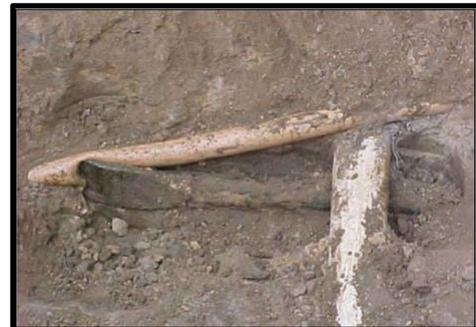
Figure 4: Class 2 Cross Bore. New communications HDD intersects sewer lateral then gas distribution line
