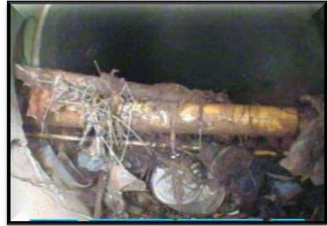
Figure 3a: Class 1 Cross bore of Gas in Sewer.
